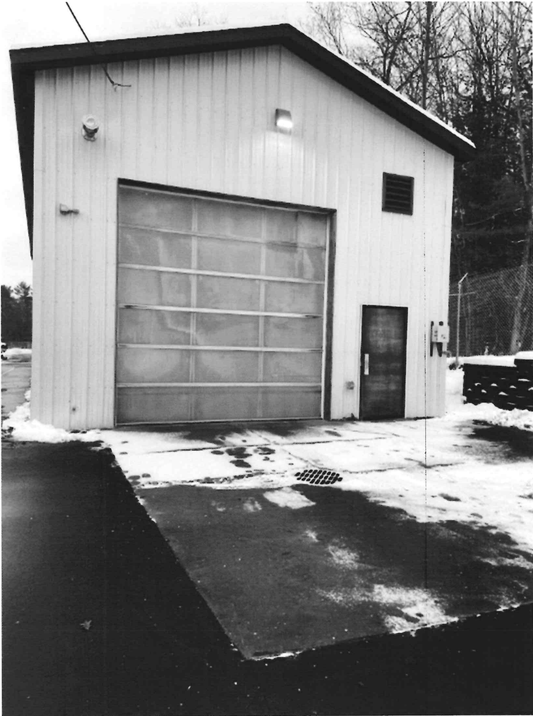
EXISTING BUS WASH BUILDING AND CONCRETE APRON
